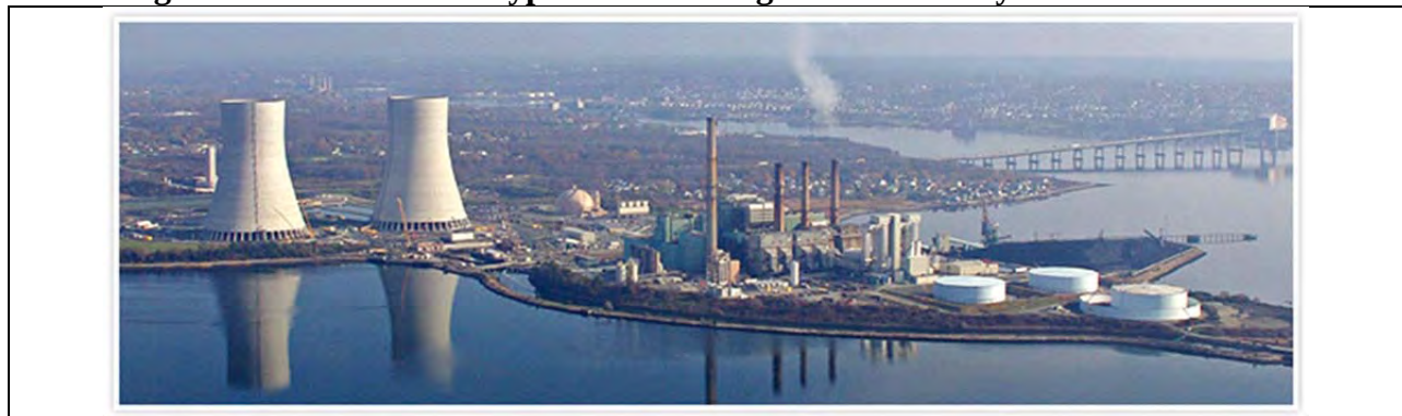
Figure 3. Natural Draft Hyperbolic Cooling Towers at Brayton Point Station 63
